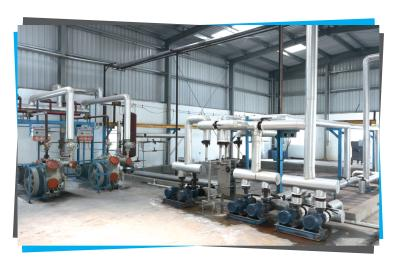
Atmospheric, PHE as well as Evaporative Condensers with in-house manufacturing capability for Atmospheric condensers, Shell and Tube Evaporators as well as Condensers.
